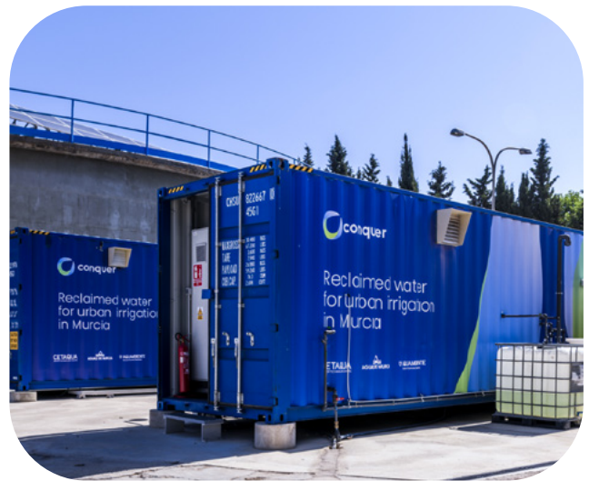
Image 1. LIFE Conquer pilot site, placed in the Zarandona water reclamation plant. Left: stage 1 (Smart NF). Right: stage 2 (Brine Valorisation).
