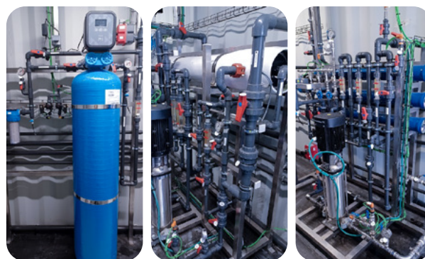
Image 3. Second-stage pretreatment train of LIFE Conquer, from left to right: ion exchange resin, nanofiltration membrane, and reverse osmosis.
