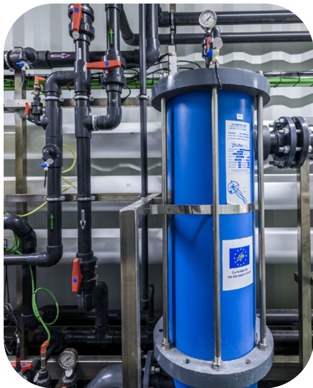
Image 2. Pre-filter (blue) of the first stage of LIFE Conquer's technology.
